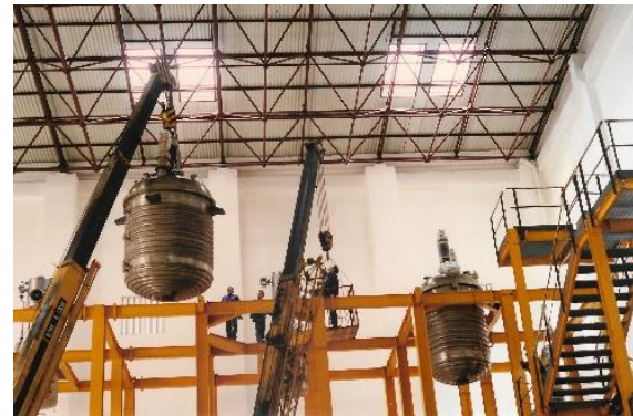
Machinery installation supervision
