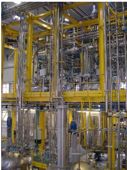
Final start-up and commissioning
